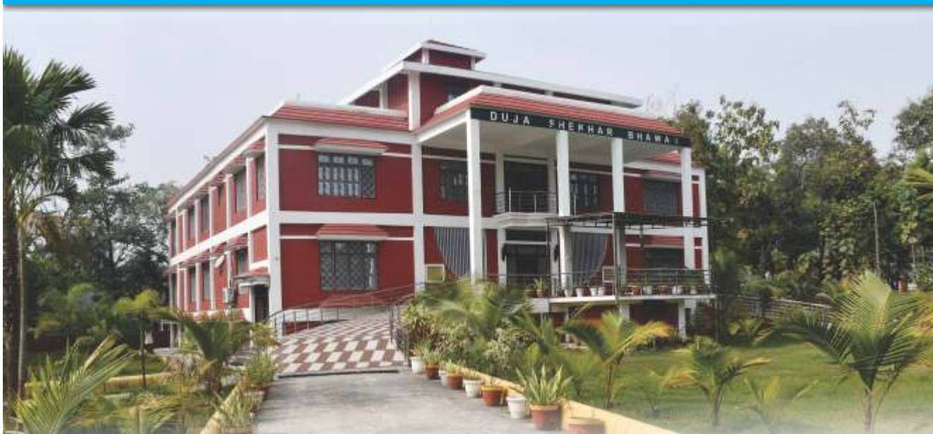
Duja Shekhar Bhawan having Library, Activity Hall, Guest House, Museum & gymnasium.
